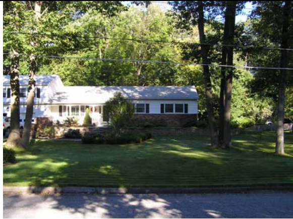
Figure 1. Front view of 14 Hearthside Drive.
