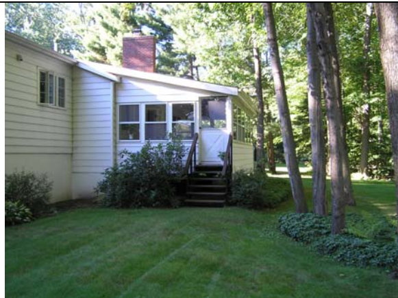
Figure 3. Our backyard showing raised deck.
