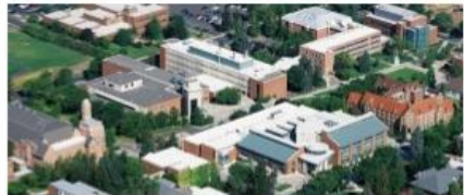
Condenser (University of Idaho Campus Steam Distribution)
