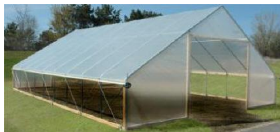
Figure 1: Demonstrating the Gothic Frame Style. Photo taken from Gothic Arch Greenhouse's Website
