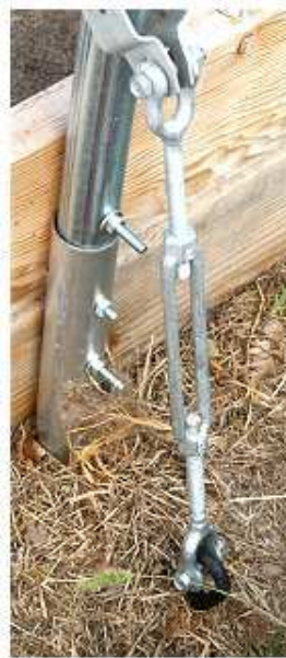
Figure 2: This figure displays an earth anchor setup.
