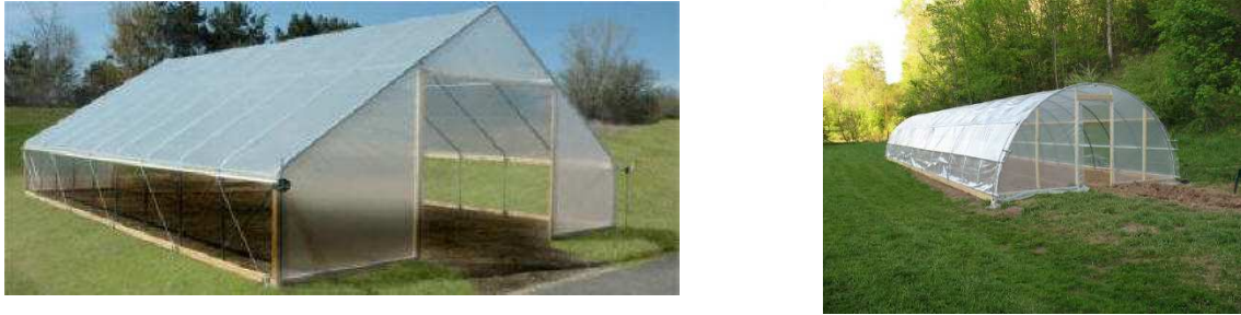
Figure 1: The left picture shows a gable style and the right shows a quonset style
