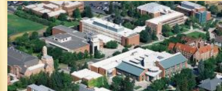
Condenser (University of Idaho Campus Steam Distribution)
