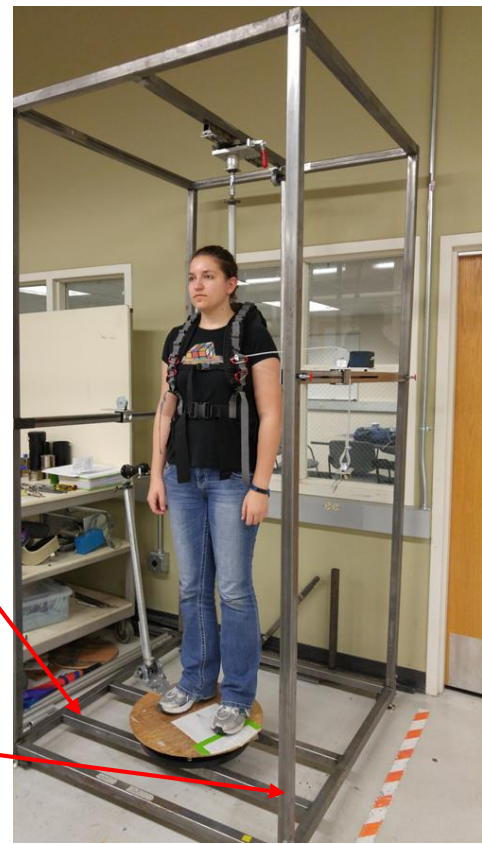
Figure 2. New Frame Construction
