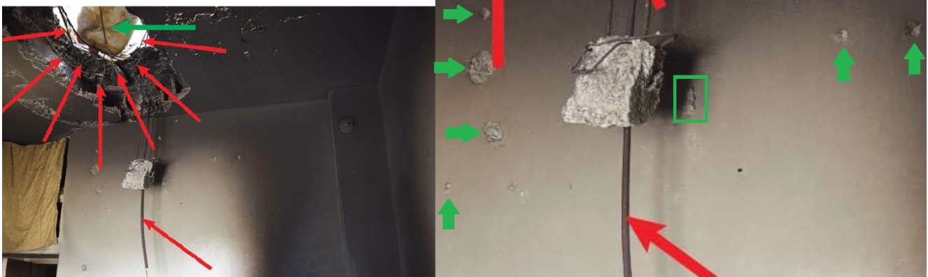
FIGURE 11: VISIBLE CRATER ON THE ROOFTOP OF LOCATION 2 PHOTOGRAPHED FROM THE ROOM DIRECTLY BELOW. PART OF THE YELLOW INDUSTRIAL CYLINDER (MARKED WITH A GREEN ARROW) AND DEPOSITS OF BLACKENING SOOT ON BOTH THE CEILING AND THE WALLS ARE VISIBLE. NO FRAGMENTATION DAMAGE PATTERN CONSISTENT WITH EXPLOSION IS VISIBLE ON THE WALLS.
